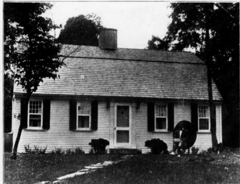
House two centuries old that was cut into sections and shipped by rail to a new location
